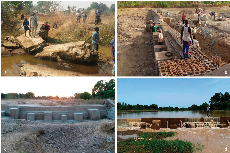
Figure 5. The rebuilding process in Toumbouba: (a) the old barrage down; (b) the building phase; (c) the wall complete; (d) the barrage working phase (Source: Authors’).
