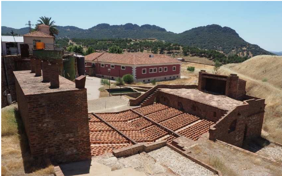
Figure 2. Buildings at the Almadén Mining Park (aludel kilns and Mercury Museum). Source: María del Carmen Cañizares Ruiz.
