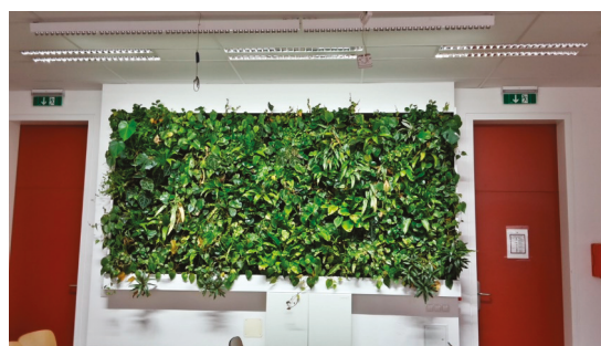
Figure 2. Fleece system in Building B.
