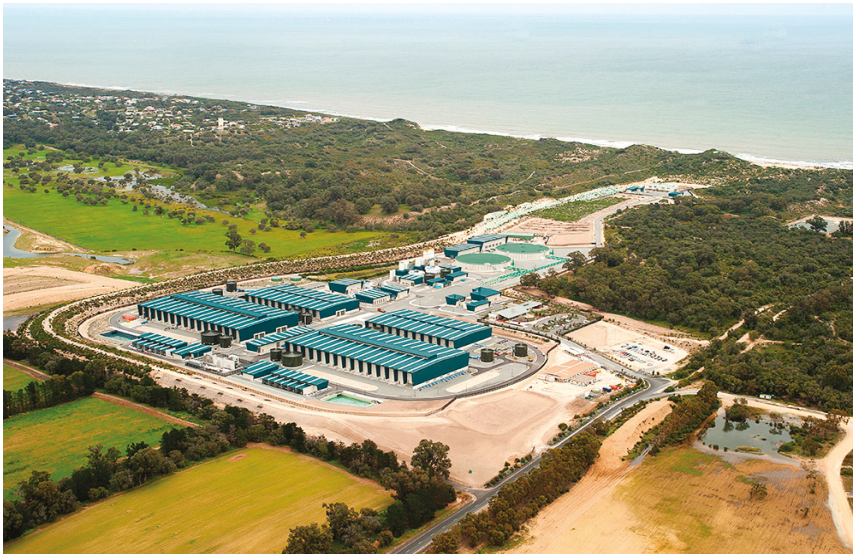
Figure 2. SSDP, general view. Source: Water Corporation.
