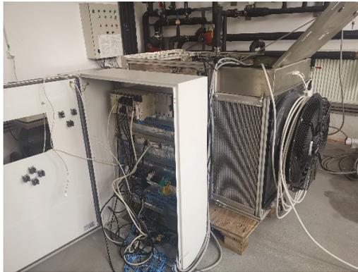
Figure 11. CPU and automation panel.
