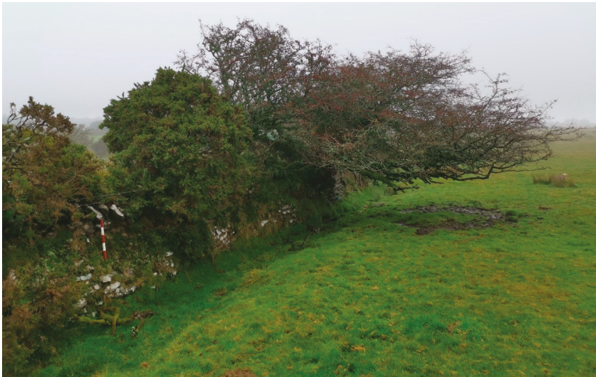
Figure 5. Dry stone sections of the Ladydown Common enclosures, in the form of a traditional Cornish Hedge. Scale 50 cm (Photograph: Richard Grove).
