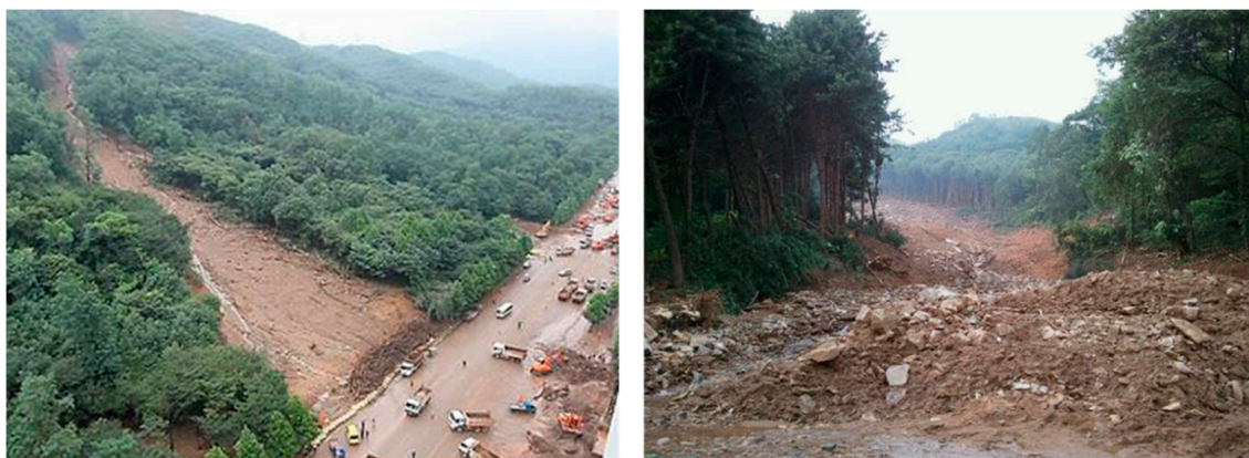
Figure 3. Landslide status on the northern side of Mt. Umyeon in 2011 [39,40].
