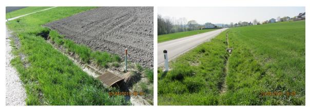
**Figure 3.** Roadside ditch with multiple storm drains at varying distances. The left picture was taken upstream of the right.
