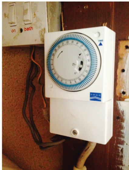
Figure 5. The interior of Joan's 'hot-press', displaying the central heating timer and immersion heater on the left, and torch on the right. Permission granted by Dr. L Shore.
