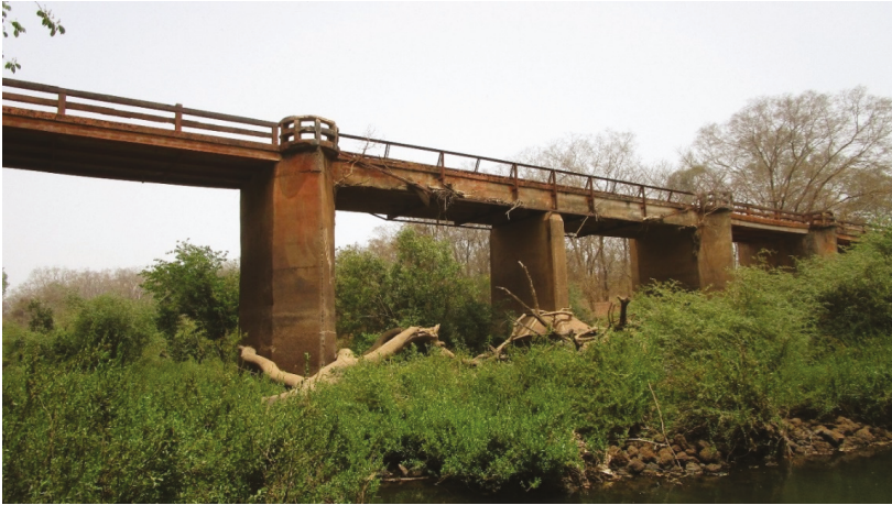
Figure 15. Bridge of the Koundara-Youkounkoun road, northern Guinea, on the Koulountou River. Built in the 1950s, it was flooded by the streamflow in August 2018, depositing whole trees (bottom) and wood debris (on the bridge deck).
