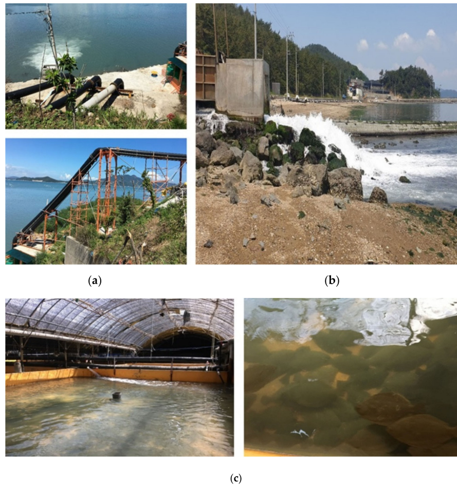
Figure 1. Fish farm facilities: (a) water supply system; (b) discharge water system; (c) fish farm.
