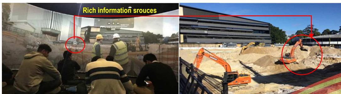
Figure 8. The immersive environment used for the case course at the University of New South Wales (UNSW) (right), A selected Hotspot Site Layout Interview—Bulk excavation (left), the produced module, including the hot spots linked to rich information for each topic.
