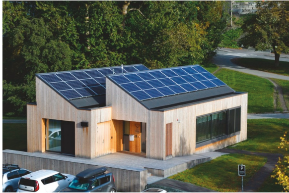
Figure 6. Building ZEB Lab provided by NTNU (Norway).
