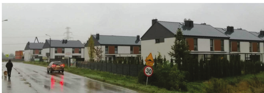
Figure 12. A typical new housing estate in the suburbs of Warsaw.
