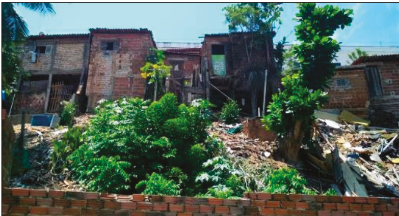
Figure 15. Waste and rubble deposition on the hillside within the site area.
