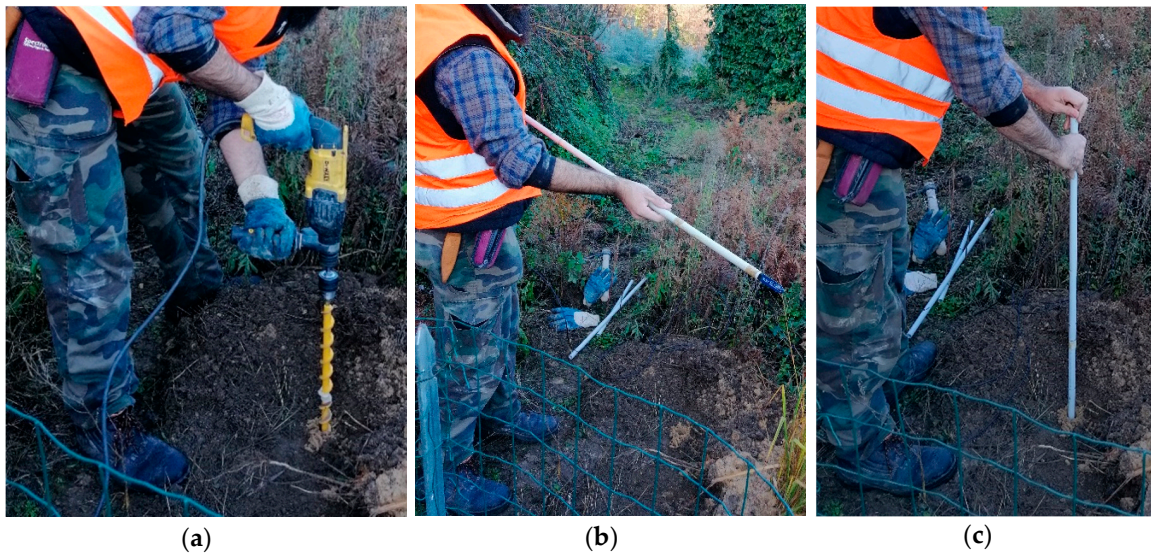
Figure 9. Vertical installation: (a) Creation of the vertical hole; (b) Positioning of the WaterScout in the PVC pipe; (c) Insertion of the sensor in the hole.
