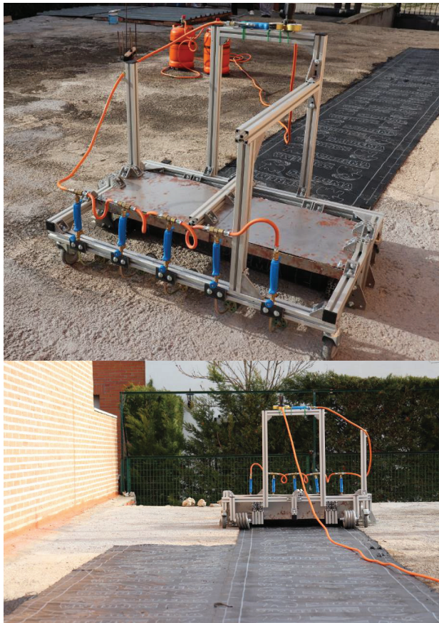
Figure 18. Asphalt rolls installation results.
