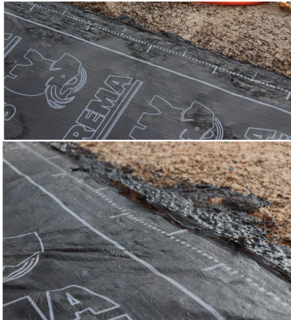
Figure 19. Quality test at overlaps.
