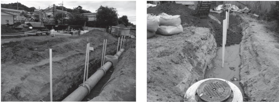
Figure 2. Backfilling of buried pipes using controlled low-strength material (CLSM) [6].
