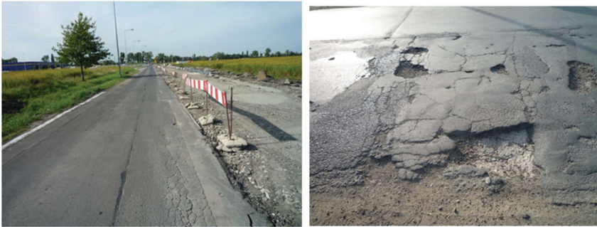
Figure 8. A section of the existing road—west lane.
