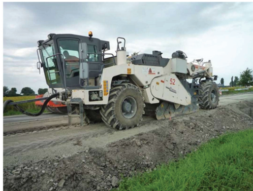
Figure 9. Recycling on-site—crushing and mixing of ingredients.
