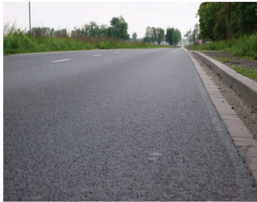
Figure 10. Wearing course layer, SMA type.
