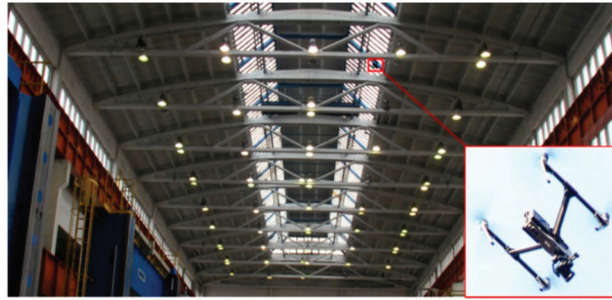
Figure 4. Visual inspection using an unmanned aerial vehicle (UAV).
