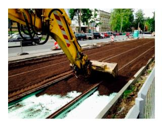
**Figure 8.** Reconstruction of a tram line—laying a lawn, Rakowiecka Street, Warsaw. Photo: J. Łukaszkiewicz, V 2015.
