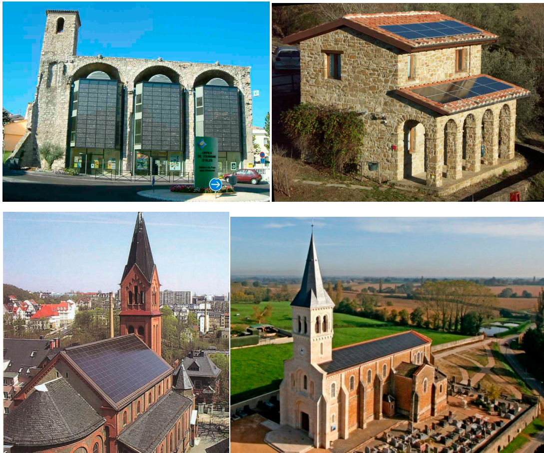
Figure 3. Implementation of somewhat controversial photovoltaic systems on heritage buildings.
