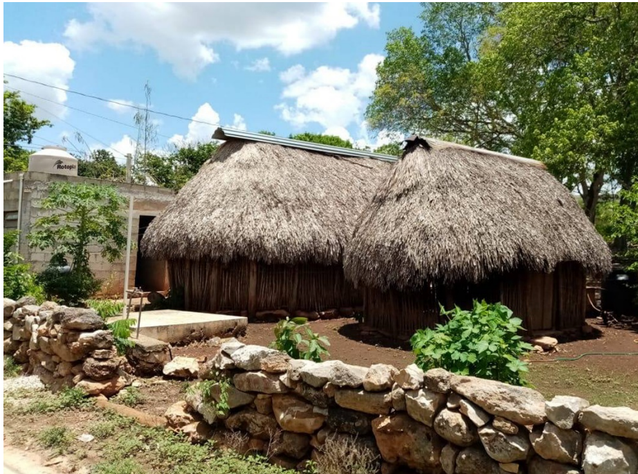
Figure 4. A cinder block house with pole and thatch auxiliary structures in Kancab.
