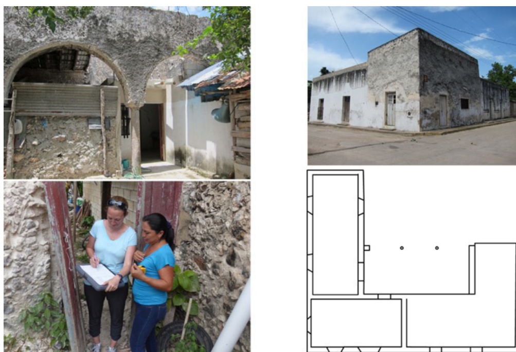
Figure 4. Documentation efforts for the colonial houses. Drawings and photographs by Kasey Diserens Morgan.
