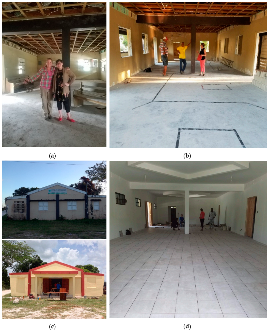
Figure 4. The renovation of the museum space in Crooked Tree during 2018: (a) Eleanor Harrison-Buck and Sara Clarke-Vivier in the space during January 2018 prior to renovation; (b) Eleanor Harrison-Buck with the village chairman and architect from Crooked Tree discussing the building design; (c) before and after shots of the building exterior; (d) Local contractors working on the building renovations.
