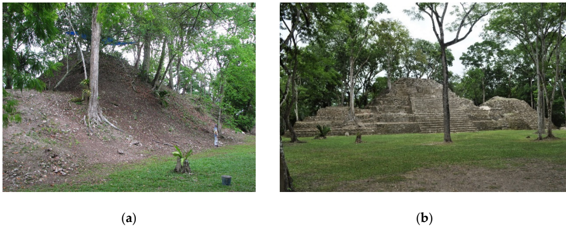
Figure 5. Photos from the conservation of the eastern triadic shrine at Cahal Pech: (a) Prior to conservation efforts (b) After conservation efforts were completed. Photos by J.J. Awe.
