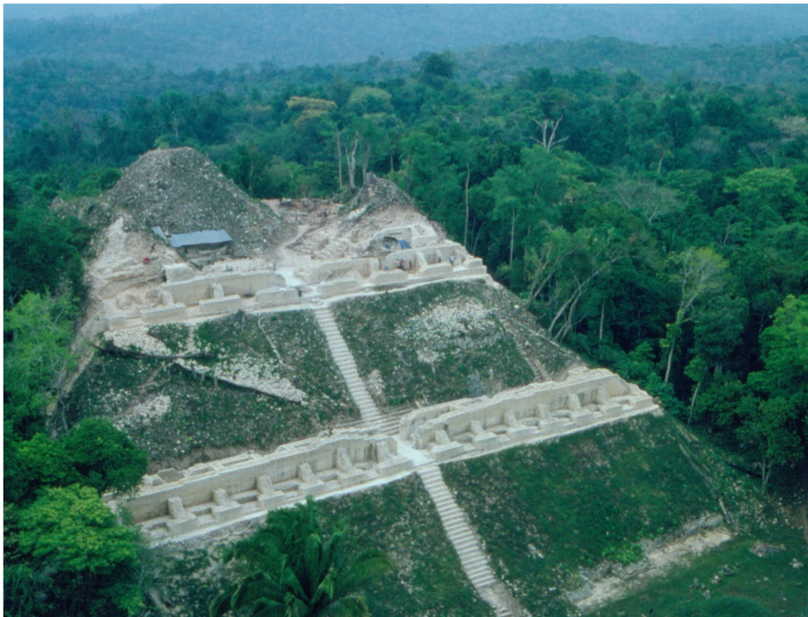
Figure 6. The USAID stabilization of the Caana architectural complex at Caracol, Belize in 1993.
