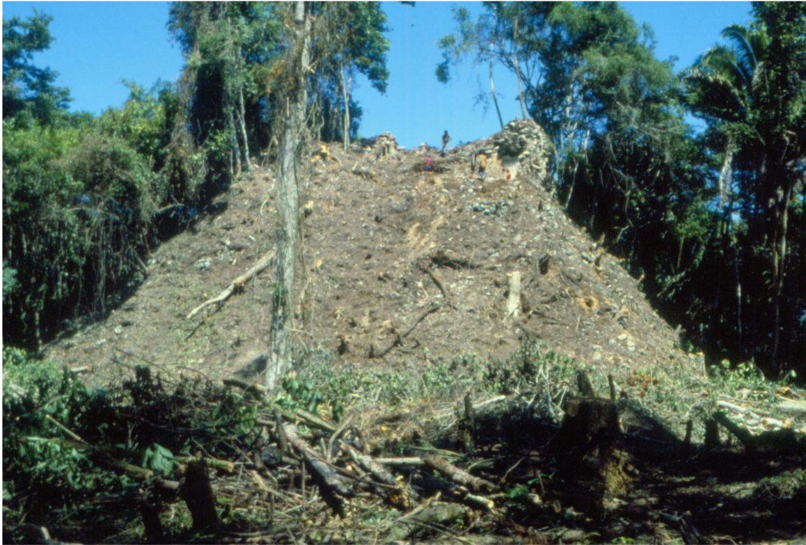
Figure 2. Caracol Structure A3 in 1986 before excavation (looking north).
