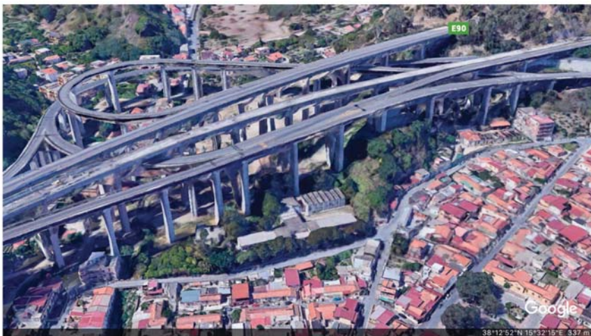
Figure 1. The "Ritiro Viaduct" in Messina (Italy).
