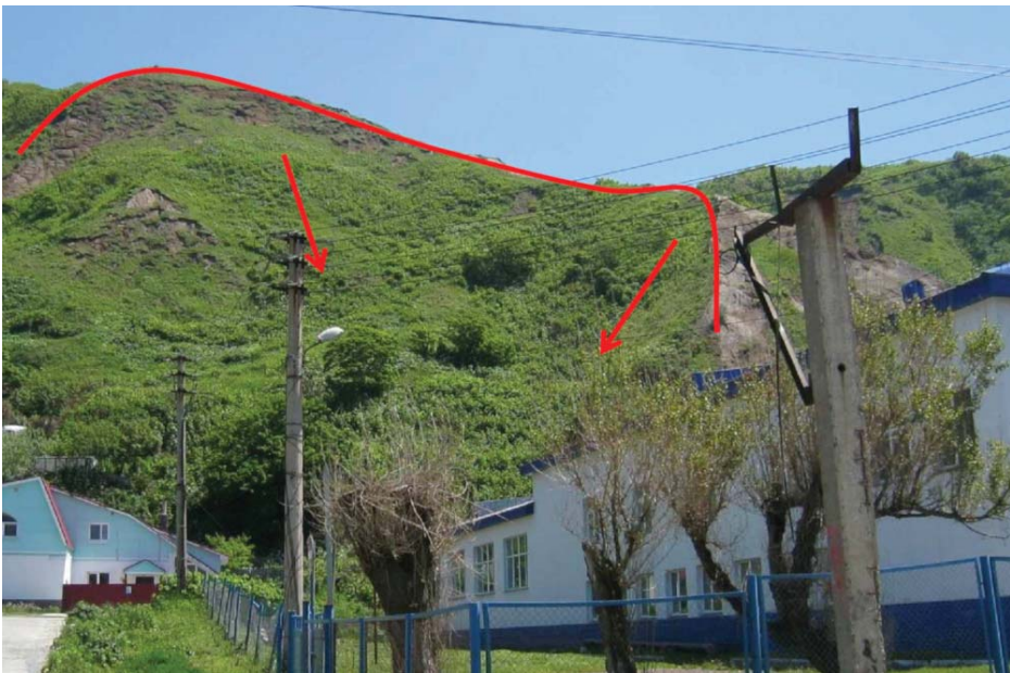
Figure 4. Side view of the location of the natural slope and school considered in this study. The red line indicates the expected landslide breakout wall. The red arrow shows the path direction of the expected landslide.
