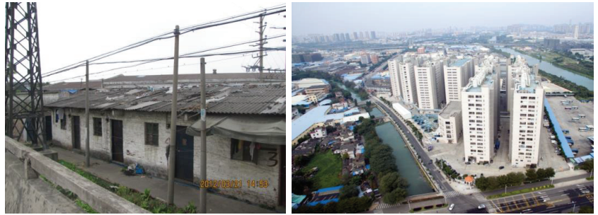
Figure 7. Before and after comparison of the renewal of Hengding Industrial Park (photo source: Urban Renewal Bureau of Shunde District).
