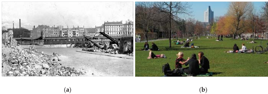
Figure 2. (a) The railway industrial area in Reudnitz [72] has been transformed into (b) the Lene-Voigt-Park (LVP) (Photo: Annegret Haase).
