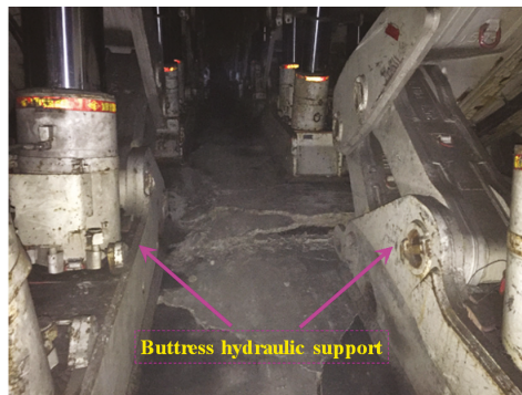
Figure 15. Photos of buttress hydraulic supports on site.
