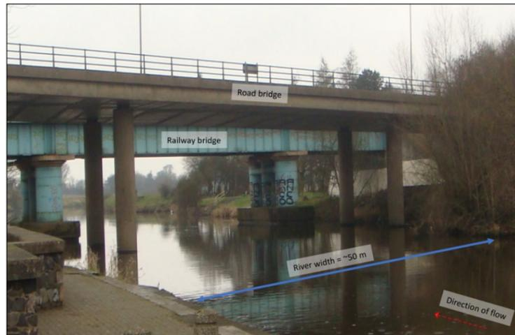
**Figure 2.** Annotated oblique view of the River Bann and the railway and road bridges studied, taken from the southwest bank (see Figure 1 for plan view map).
