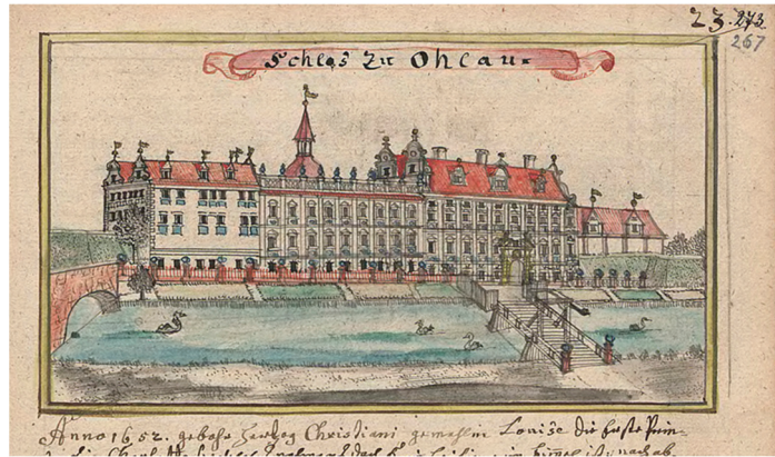
Figure 2. The southern elevation of Ohlau Castle on a drawing by F.B. Wernher from around 1730 [11] (p. 267).
