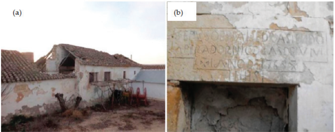
Figure 12. (a) State of the roof, partially torn down, of the “Lagar de Las Monjas” in Montilla (Córdoba) [43]; (b) lintelled stone signed by the implementer in the year 1769 in the mill of the “Lagar de las Monjas” [43].
