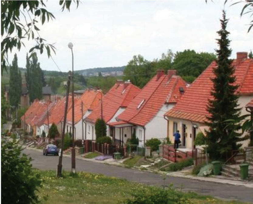
Figure 6. View of Kresowa Street in Sobiecin (Nieder Hermsdorf). Photo by the author in 2010.
