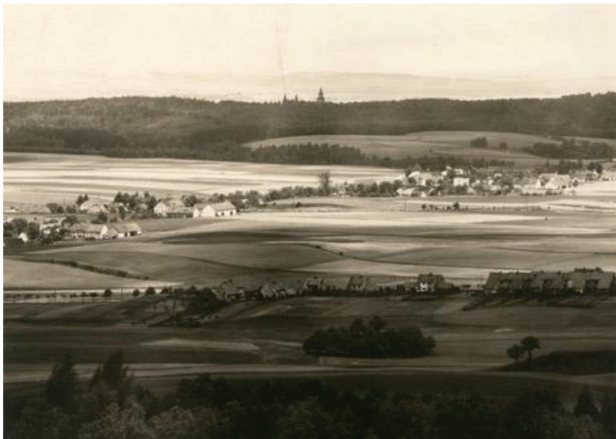
Figure 8. View of settlement on Sandberg (Piaskowa Góra) and Salzbrunn (Szcawno) in the interwar period. Adapted with permission from collection of Historical Department of the Museum in Wałbrzych (Muzeum w Wałbrzychu, Oddział Historyczny) 2877.
