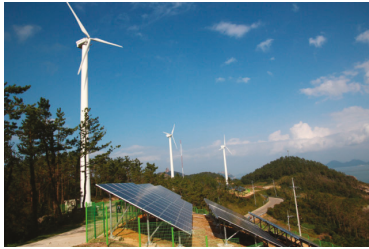
Figure 4. Wind and solar farm.
