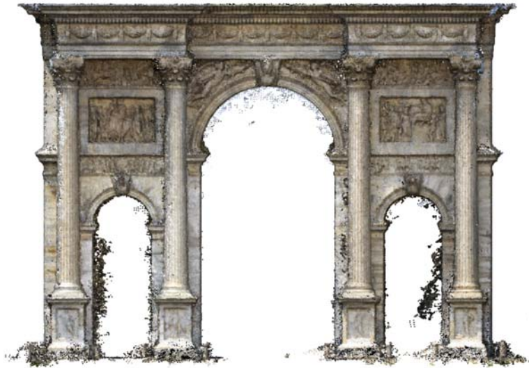
Figure 12. North elevation of the arch, terrestrial photogrammetric point cloud.
