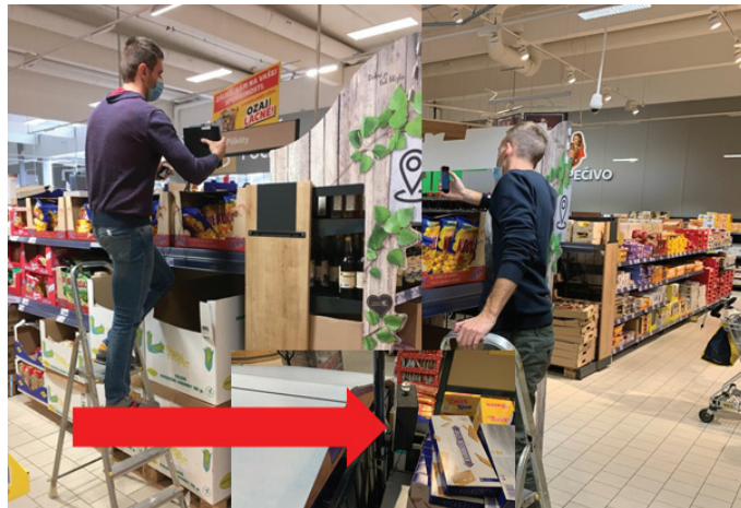
Figure 2. Installation of aromatising units in retail outlet.
