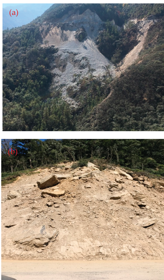
Figure 2. Landslide damages (a) near Chukha Dzongkhag (b) along the Phuentsholing–Thimphu highway.
