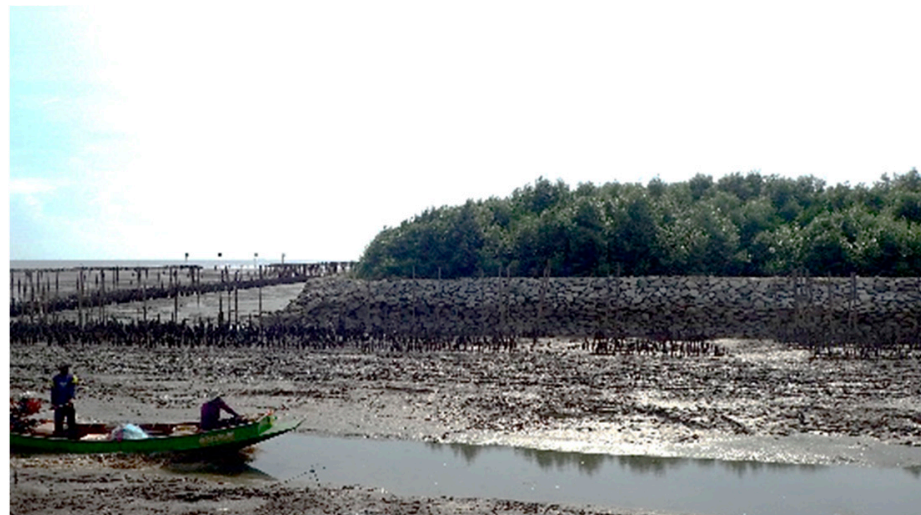
Figure 1. Successful mangrove plantation in Chonburi, Thailand—however, the rubble dike stopped the expansion of the forest [photo taken by one of the authors].
