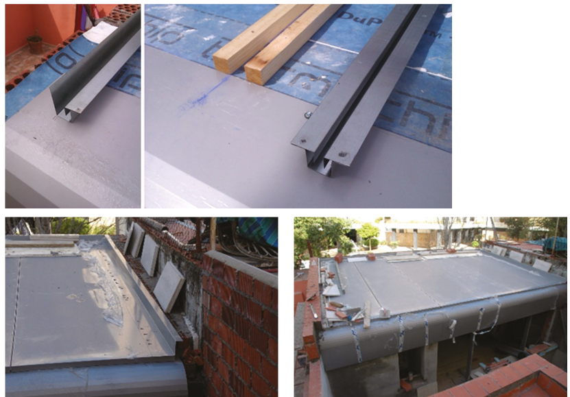
Figure 15. Side edge and centre guides. Assembly process of the coating sheets. Factory-edged finish. Photographs: authors.
