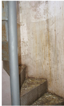
Figure 11. Stairs access to the bell tower.
