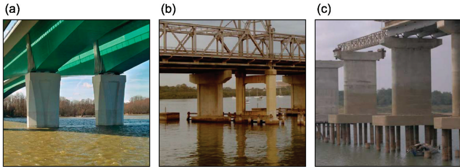
Figure 1. Typical cases of complex bridge piers in close proximity: (a) Maria Skłodowska-Curie Bridge in Warsaw, Poland; (b) Ryde Bridge in Sydney, Australia; (c) Unknown bridge under construction. (Photos from internet).
