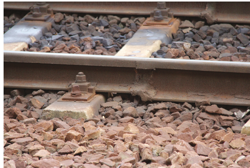
Figure 7. Thermite weld joining two rails with different profiles (50E5, UNI-50, on the right and 60E1, UNI-60, on the left).
