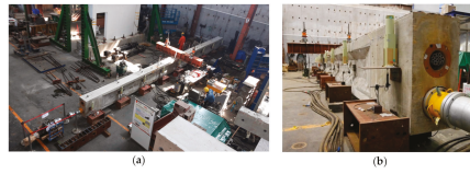
Figure 3. Three-point bending tests on a PCI girder conducted in the laboratory of NCREE, Taiwan [50]: (a) indoor test rig; (b) application of a FBG-Differential Settlement Measurement (DSM) liquid-level system for vertical deflection measurements along the span. Copyright © 2019 Elsevier Ltd. Adapted with permission.
