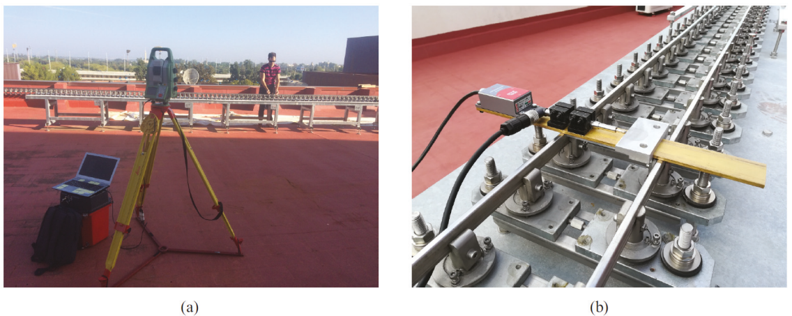
Figure 15. Irregularity measurement. (a) Robotic total station, (b) LVDT and inclinometer.
