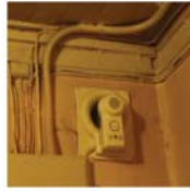
Figure 13. Integrated humidity control, occupancy sensor, and downtime (NTNU).
