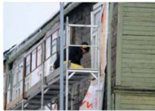
Figure 8. Renovation of the façade (Trondheim Municipality, 2016).
