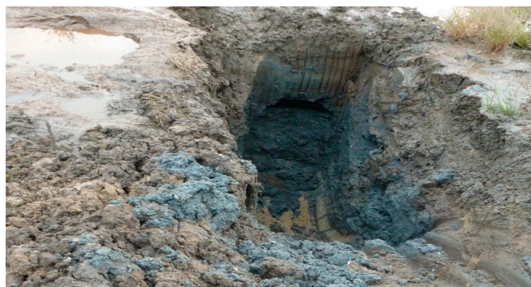
Figure 7. Site excavation of marine soft soil.
