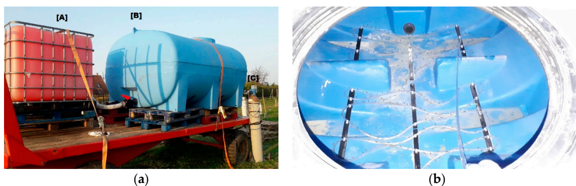
Figure 8. Views of the two tanks and the helium saturation device: (a) View of the 1 m 3 tracers tank [A], the 5 m 3 He saturated tank [B] and the compressed He cylinder [C]; (b) View from the manhole of the bubbling device in the 5 m 3 He tank (20 m of PVC pipe pierced with 200 needles of 0.5 mm diameter).
