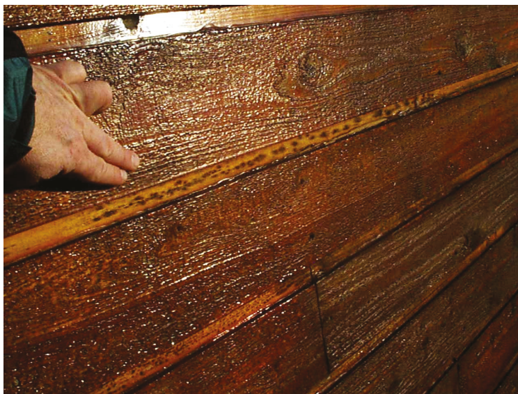
Figure 4. An example of fungal growth that has developed underneath a coating film (on the wood strip below hand) by penetrating the coating surface. This type of fungal attack occurs with opaque coatings as well, but it is readily observed when clear-polymer coatings are attacked. Clear coatings typically lack adequate UV resistance leading to development of micro-cracks in the coatings that fungi can exploit. (Goodell photo).
