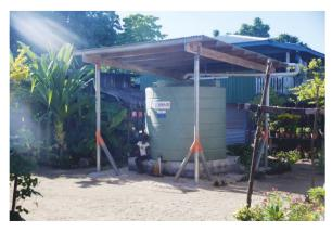
Figure 11. Rainwater storage tank on Kwai Island (J. van der Ploeg, 2017).
