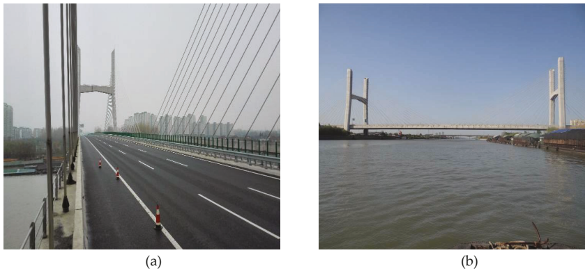
Figure 8. The Grand Canal Bridge: (a) bridge deck; (b) whole bridge.
