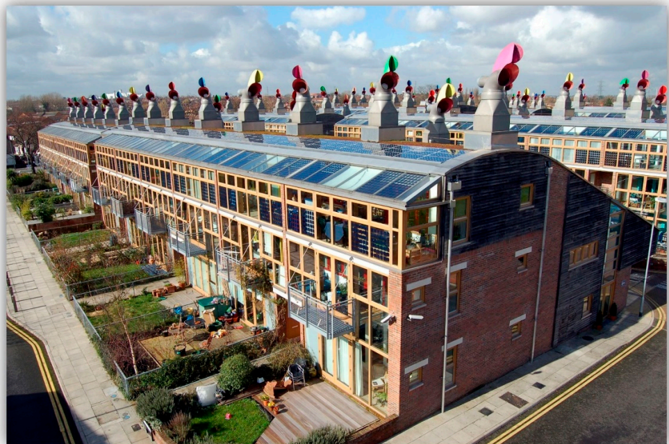
Figure 1. BedZED project in Hackbridge, London borough of Sutton, with solar panels, wind cowls, and green roofs. Source: Image credits Tom Chance https://www.flickr.com/photos/tomchance/1008213420/ CC BY 2.0, accessed on 22 July 2021.
