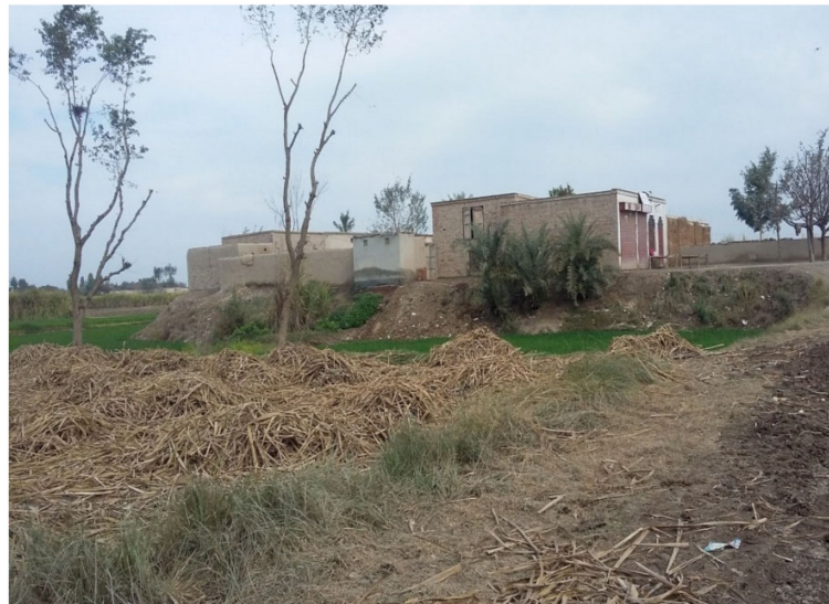
Figure 16. Practice of raised plinth level in flood-prone communities of LN, district Layyah.
