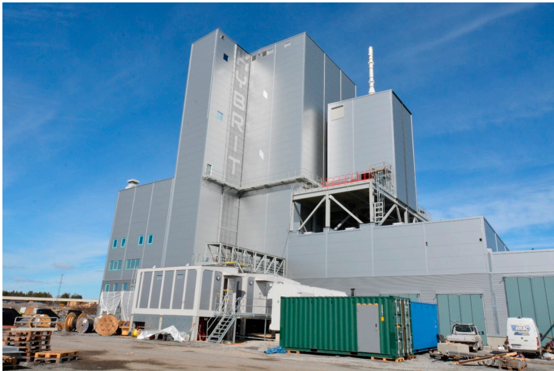
Figure 8. The pilot plant in Luleå, Sweden, under construction.
