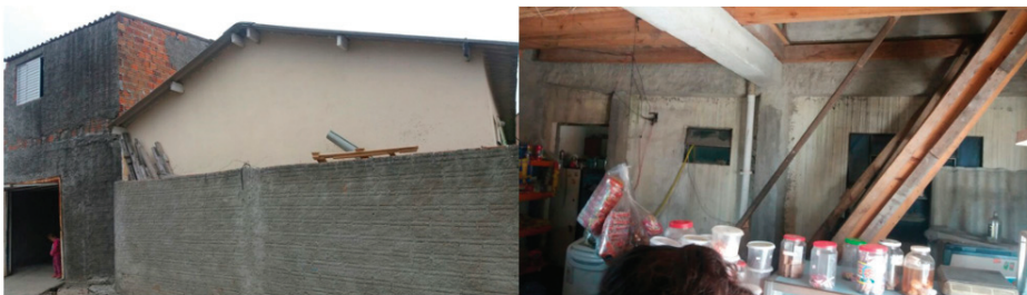
Figure 5. Example of housing unit with expansions. Images courtesy of NAUrb-UFPeL [21].
