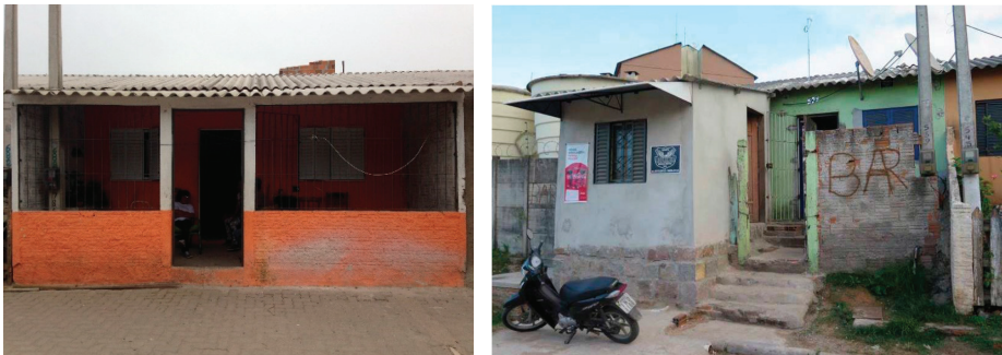
Figure 3. Example of expansions encroaching onto the public space. Images courtesy of NAUrb-UFPel [21].
