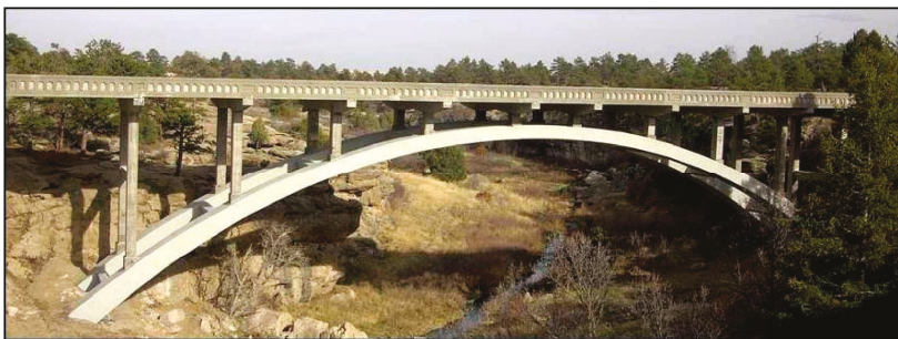
Figure 2. Castlewood Canyon bridge, Franktown, Colorado.
