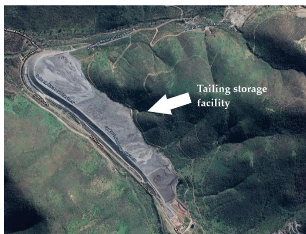
Figure 1. Tailing storage facility (32°28′16.1″ S, 71°05′00.2″ W).
