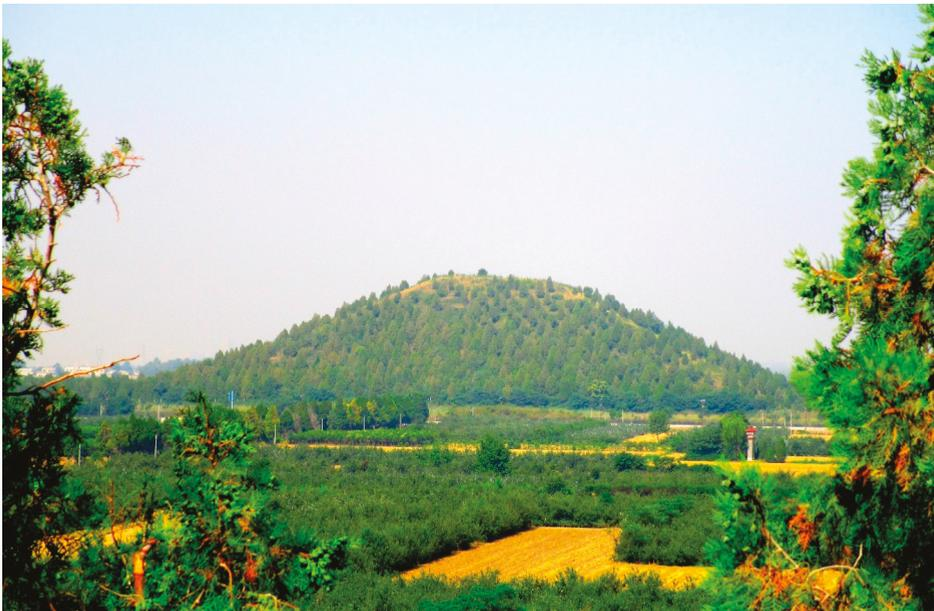
**Figure 2.** The huge burial mound of Maoling, the tomb of emperor Wu of Han, looks like a smoothed, natural hill. It is, instead, fully artificial: a pyramid made of hard rammed earth. (Photograph by the author.)
