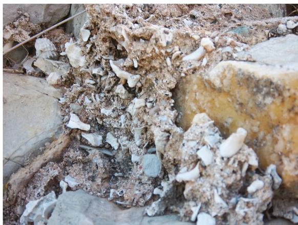
**Figure 8.** Murex shells used as binder in the wall of Hermione, next to the Bisti area where the famous local dyeing workshops were located (photograph by V. Gatsos).
