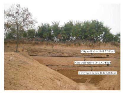
Figure 9. Cross-section showing the chronological sequence of walls in Kaifeng. (Author's photograph, 2014.).
