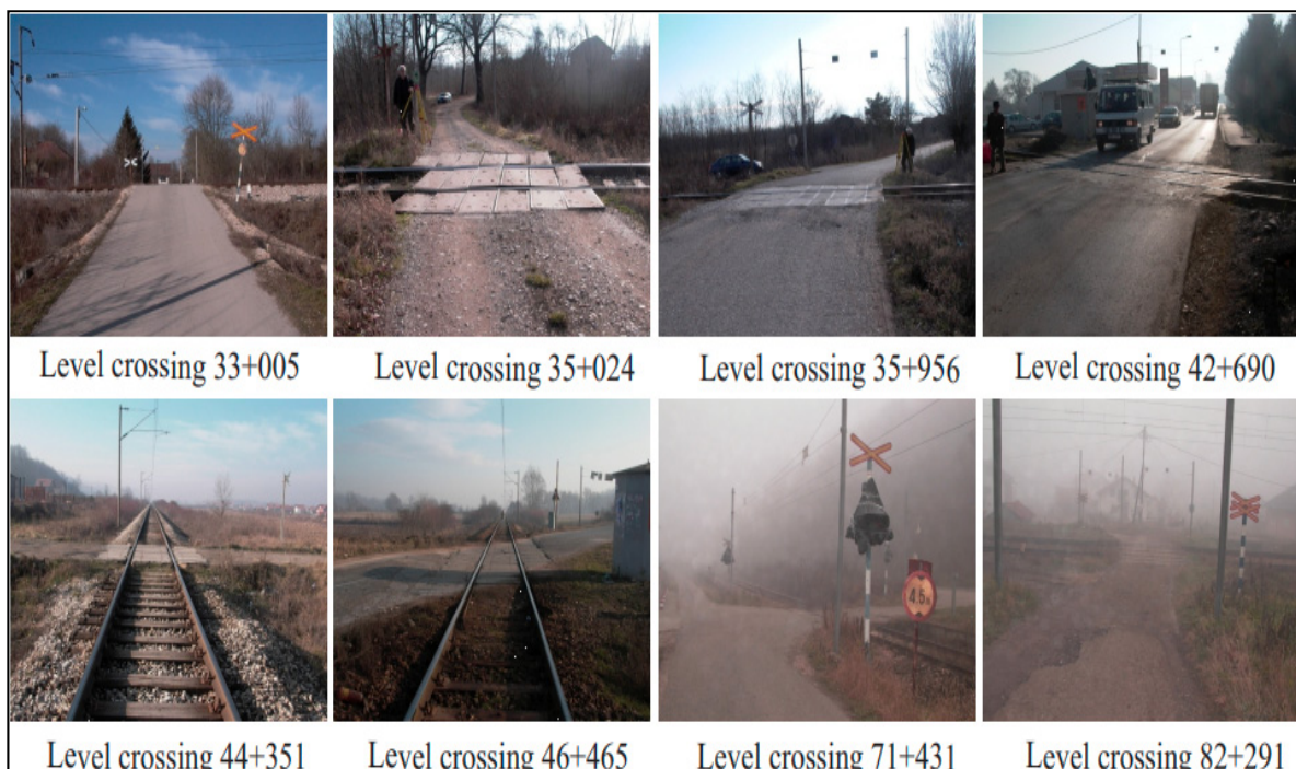
Figure 3. Overview of level crossings considered in the multi-criteria decision-making (MCDM) model.
